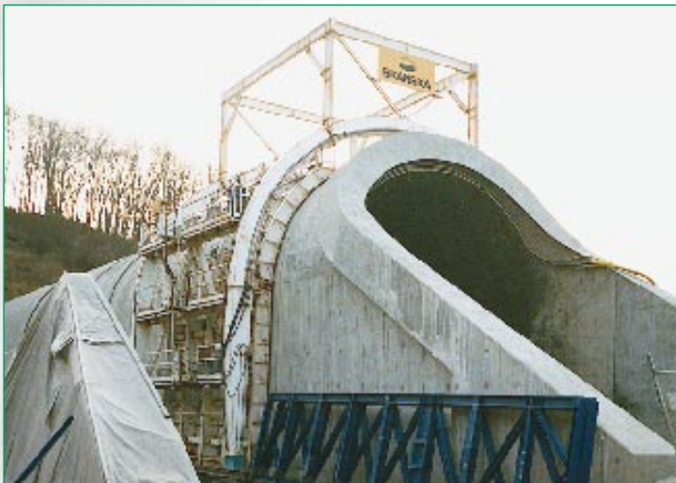
The insertion structure of the Hallandsås tunnel.
